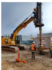
Drilling for Canopy Structure
