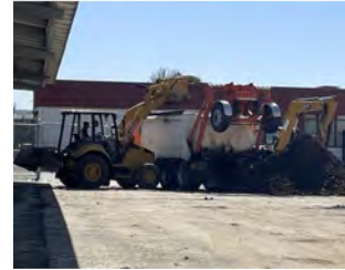
Removing Soil Stockpiles
