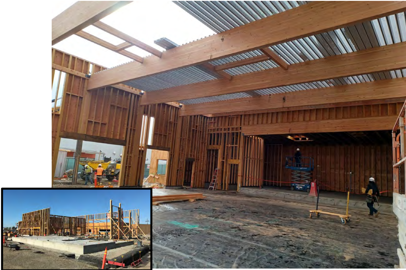
Multi-Purpose Room wall framing is complete
