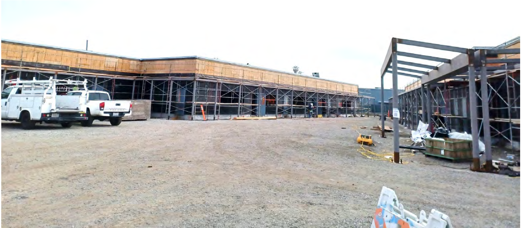
Building F and E - Preparing for stucco
